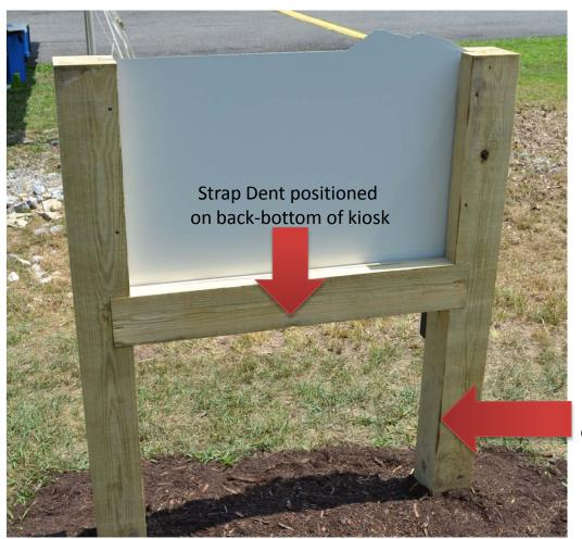
Slivered edge positioned on back-inside edge of kiosk
