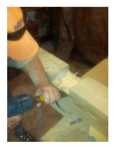
Use your hands to break out the majority of the wood slices. The use a chisel to clean up the rest and smooth out the notch.
