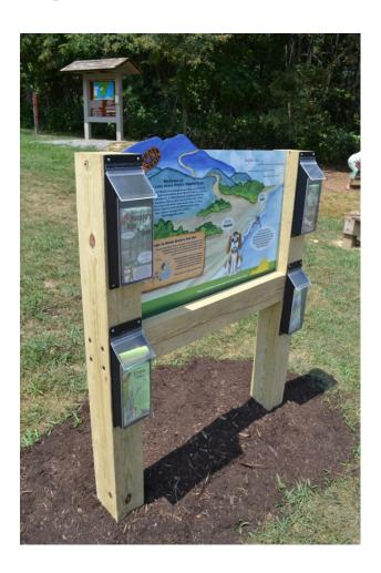
Install the sign so that the top of the sign is aligned with the top of the 6x6's on their inside edge. Make sure the sign is level. Install the brochure boxes at reasonable heights for ease of use.
