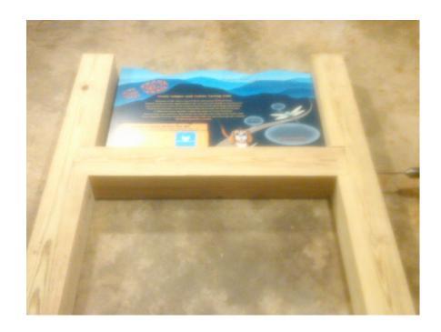
If you have the sign available, do a dry fit of the sign to ensure that the sign slides into the channel properly. If the channel is out of line, the sign will not fit. However, for added protection of the sign itself, do not permanently install the sign until the kiosk is ready to be installed in the ground.
