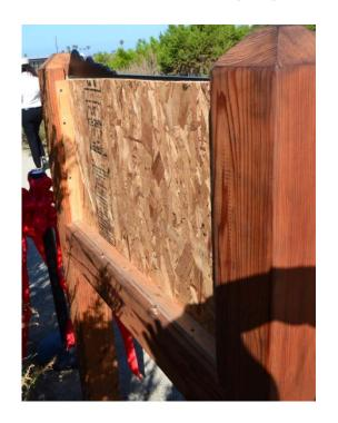
Install a  $36'' \times 20''$  piece of 1/2'' plywood to help support the back of the sign.
