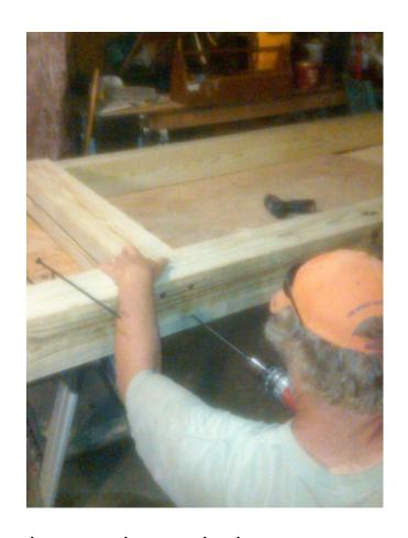
Use 12" long (or longer) Lag Screws to anchor the cross bar to the legs. Install 3-4 lag screws on each side, avoiding the channel.
